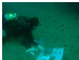
Fig (37) painting process under water
